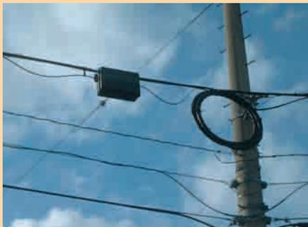
*Distribution box for fiber lashed to existing aerial cable; this method is quick and inexpensive.*
